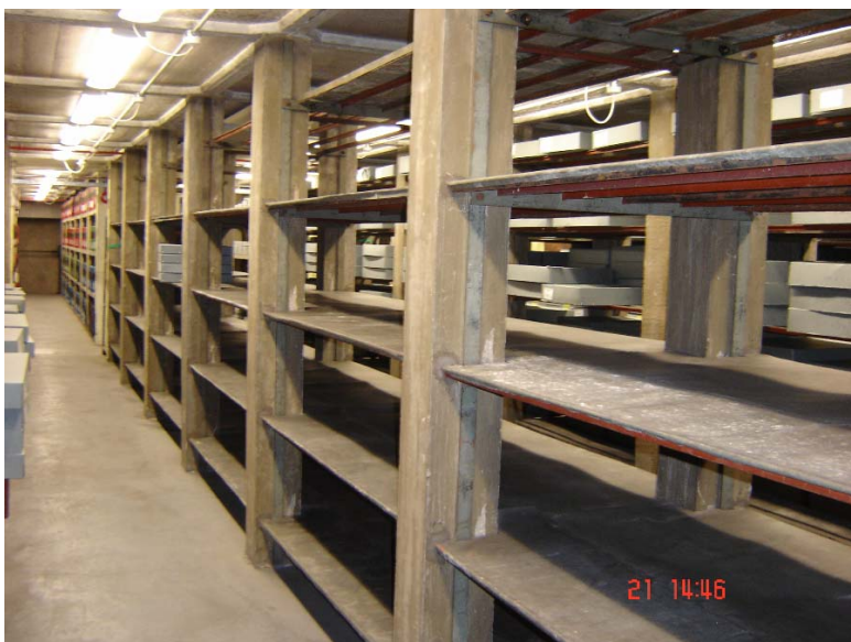
Room 2C in the Four Courts. Steel shelving welded into concrete pillars was replaced with modern static shelving.
